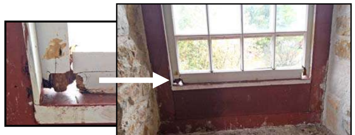
Daylight showing through a rotted out window sash in the Old Stone Mill (close up on left)
