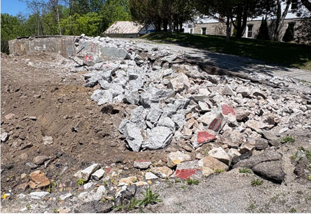
Remaining foundation east property line
