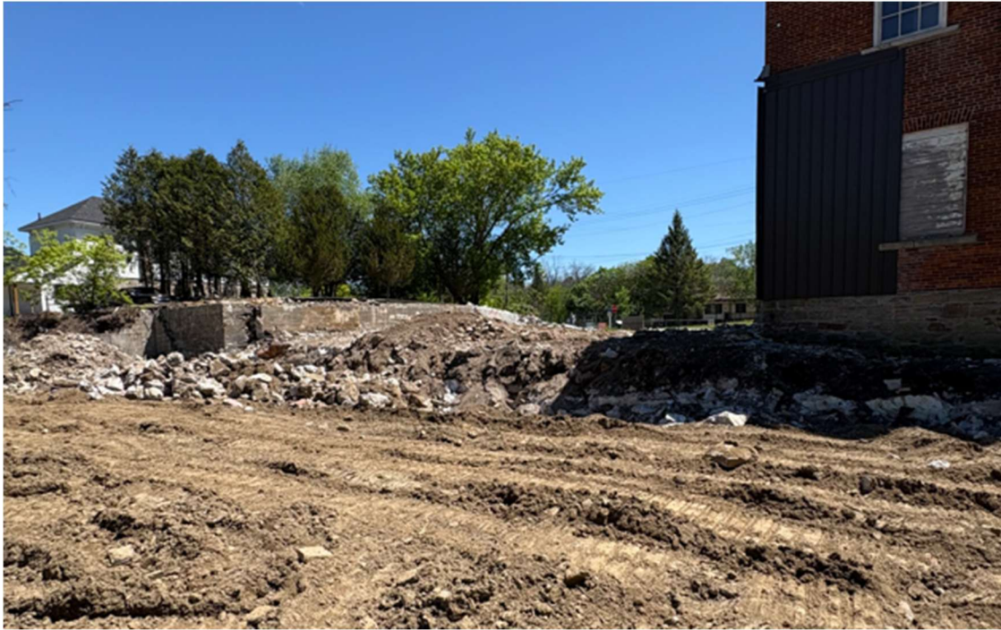
View of the west of foundation at retaining wall
