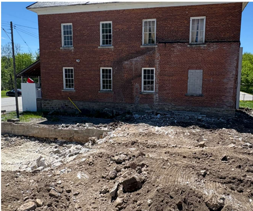
South Old Town Hall remaining foundation
