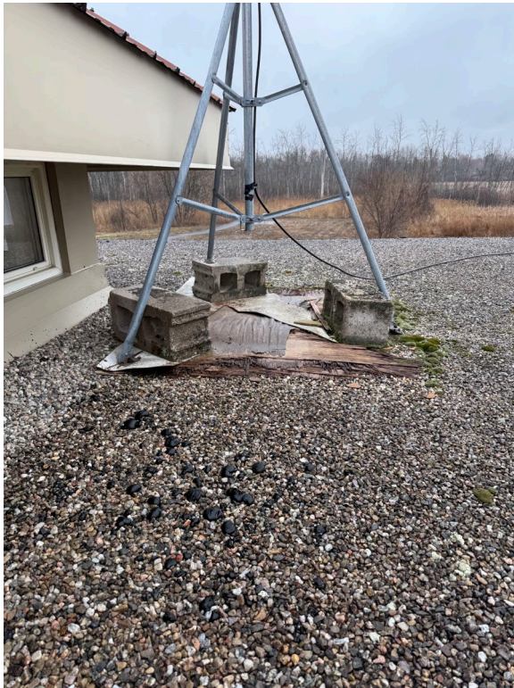
VIEW OF BALLASTED ANTENNA TO BE REMOVED & DISPOSED
