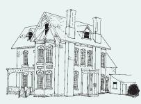
constructed with detail of Gothic Revival style. It is an extraordinarily tall building, being some two-and-one-half storeys. The 1<sup>st</sup> storey was constructed of 5 courses of brick, the 2<sup>nd,</sup> four courses and the 3<sup>rd</sup> of three, with inner walls of lath and plaster. To offset this dramatic perception of height, a two-storey bay extends from the front wing. Extensive
