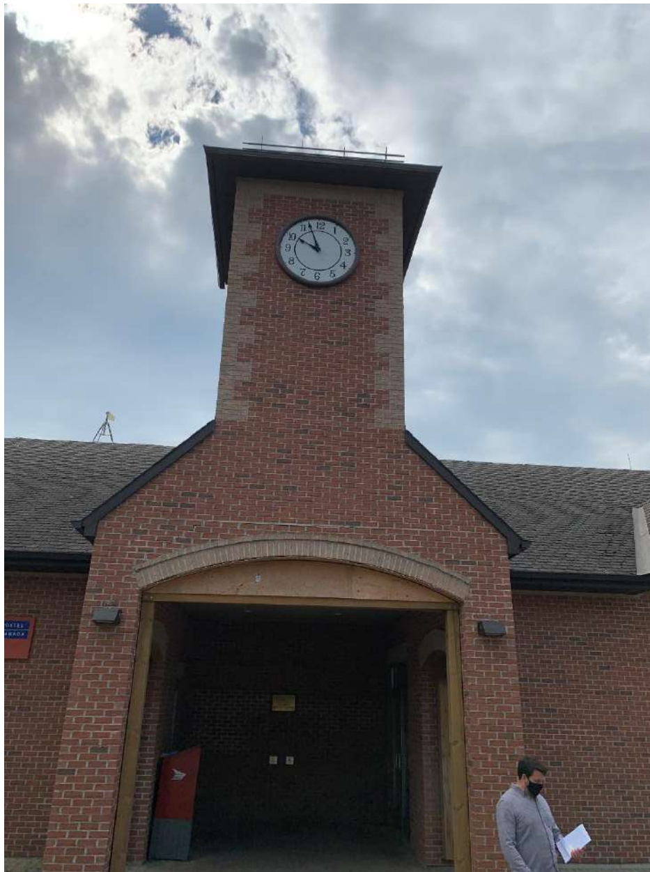
Figure 2: Overall view of tower.
