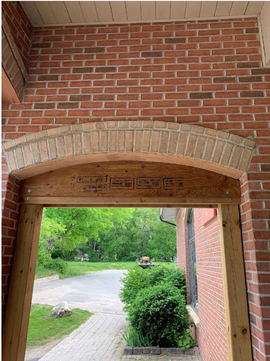
Figure 6: Side arch from inside.
