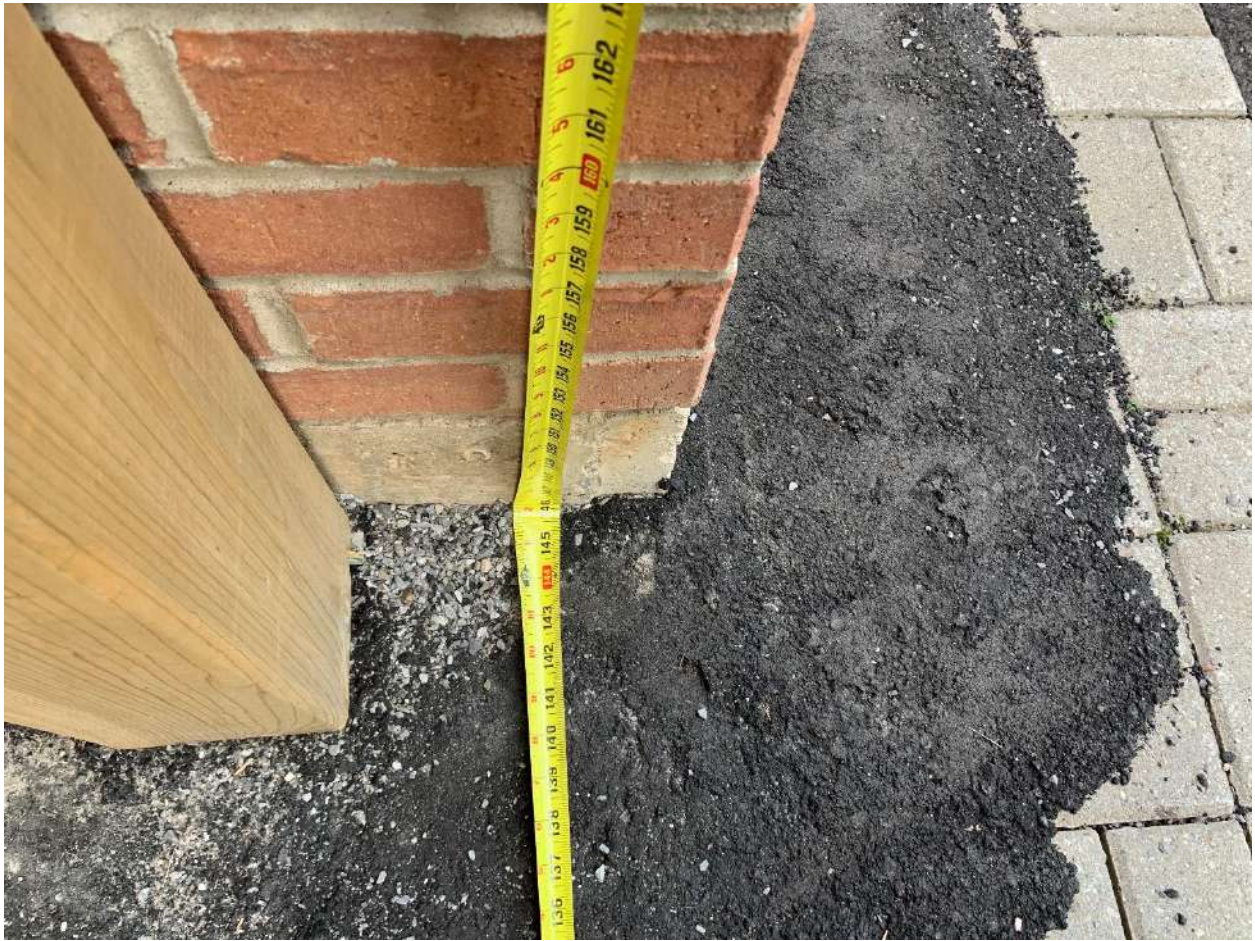
Figure 17: Brick pier at base.
