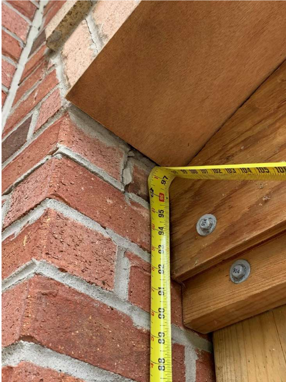
Figure 12: Cracked mortar
