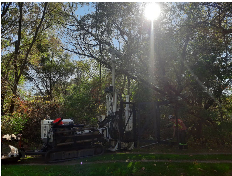
Photo 3 Drilling BH102, October 2023.
