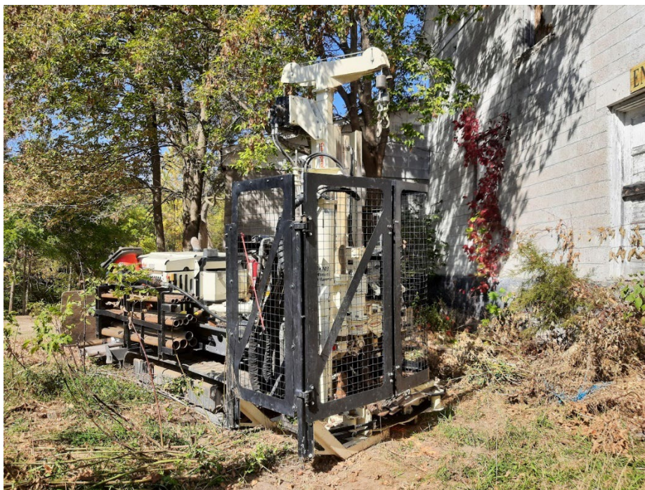
Photo 5 Set up – BH104, October 2023.
