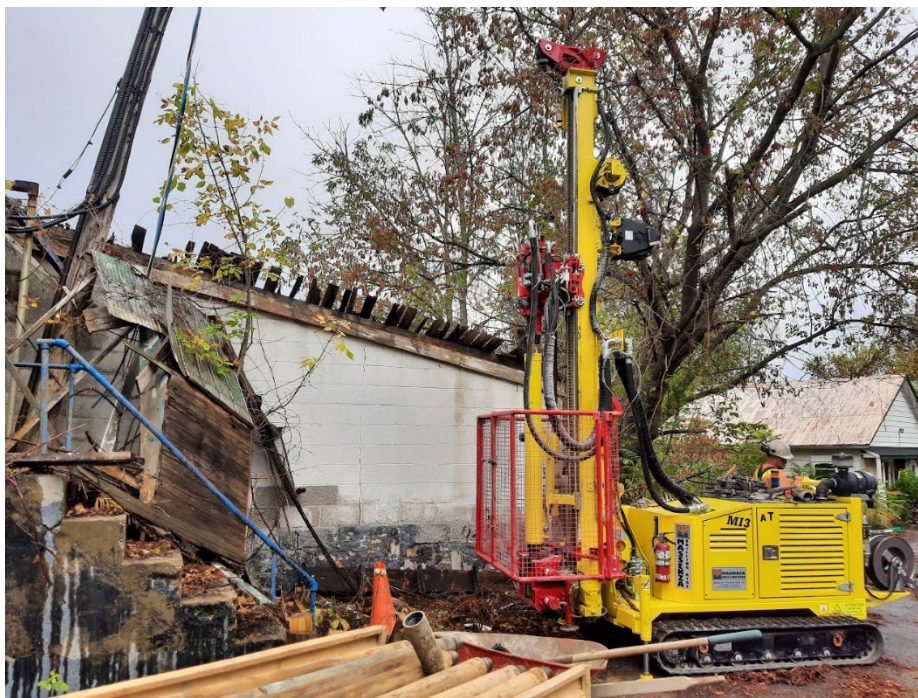
Photo 13 Drilling BH109, October 2023.
