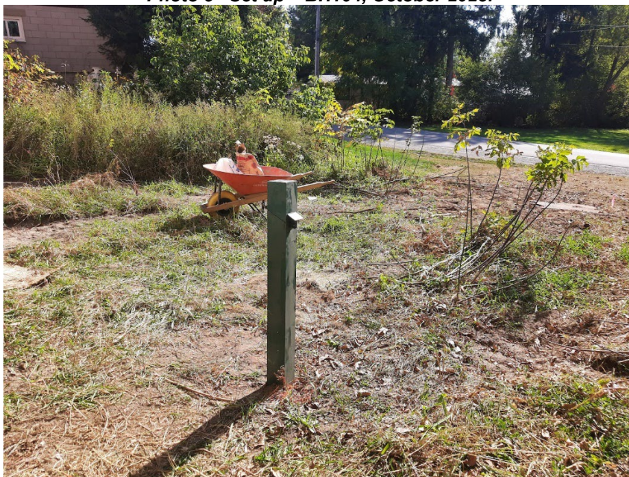
Photo 6 BH104 completed with monitoring well, October 2023.
