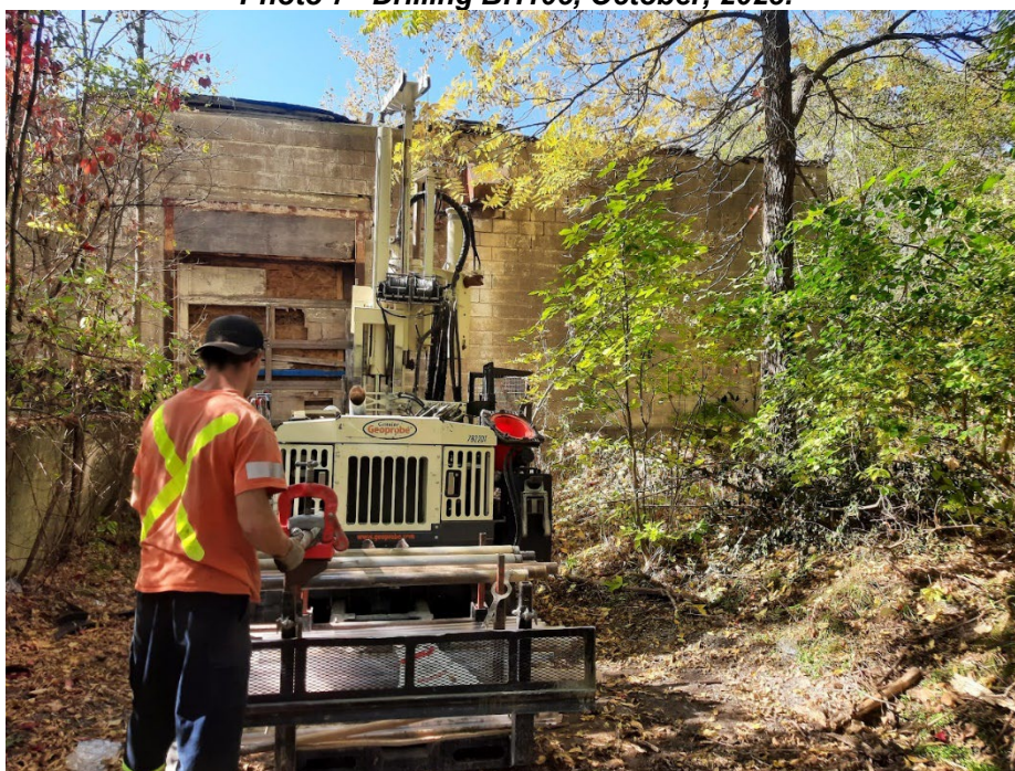
Photo 8 Drilling BH106, October 2023.
