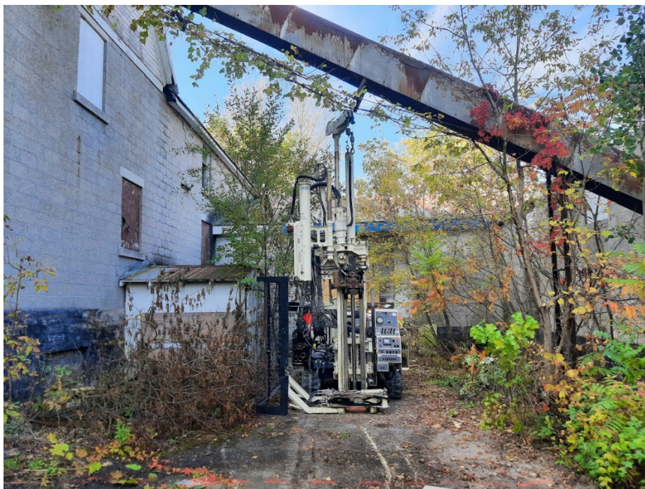
Photo 7 Drilling BH105, October, 2023.
