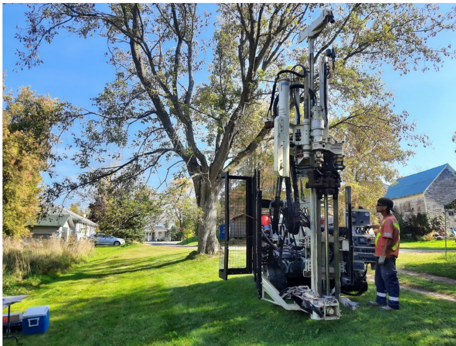
Photo 1 Drilling BH101, October 2023.
