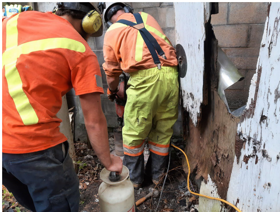
Photo 11 Coring BH108, October 2023.
