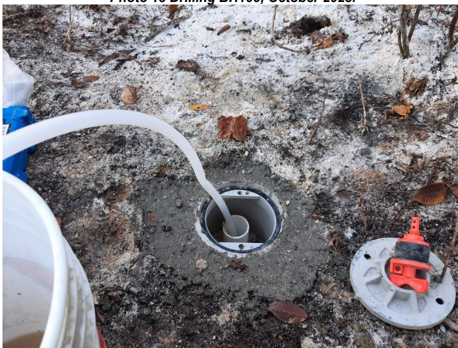
Photo 14 BH109 completed with a monitoring well, October 2023.
