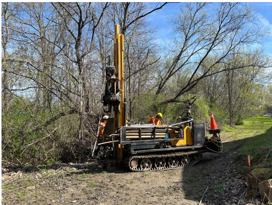
Photo 15 Drilling BH201, May 2024.
