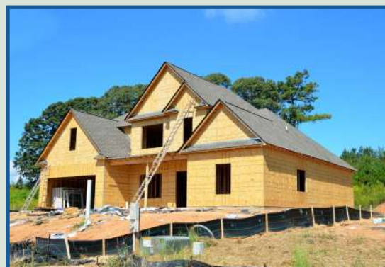
The above photo shows an example of silt fencing used during development to keep sediment of construction away from other features on the property.
